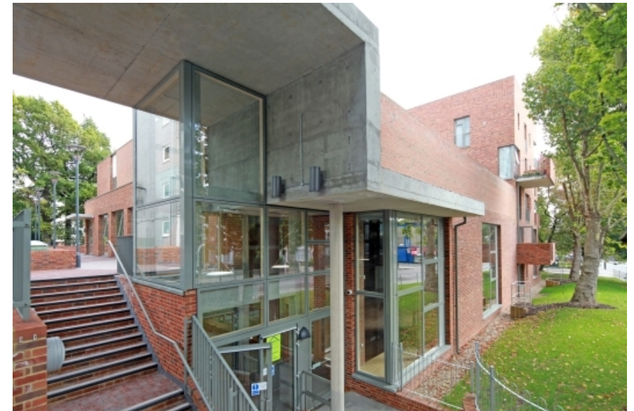
Holly Park / Brickworks
